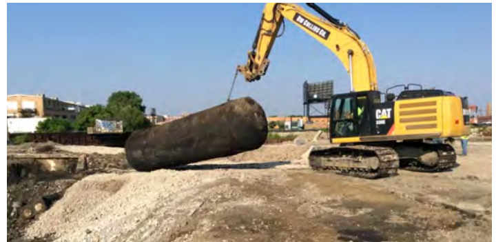
A tank containing petroleum products is removed from the site. Photo by V3 Companies, courtesy Sterling Bay
