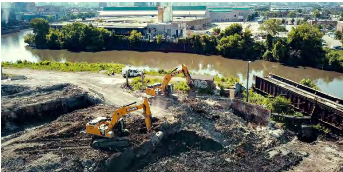
Before work can begin on Chicago's $6 billion Lincoln Yards, crews must complete a major cleanup. (R W Collins photo)
